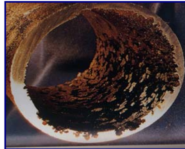
Under Deposit Corrosion View after Cleaning
